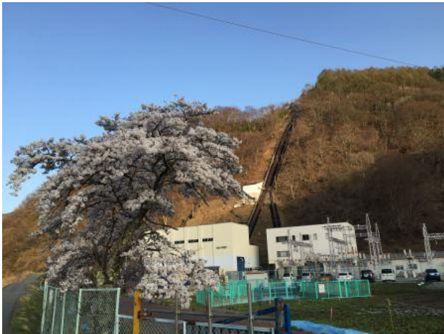
Exterior of Mibugawa No. 1 Power Station
