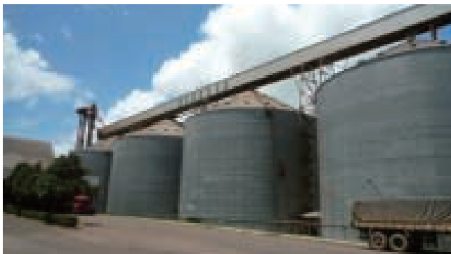
A grain storage facility in Brazil.
