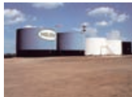
Fertilizer storage tank owned by Helena Chemical , U.S.A
