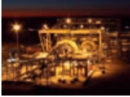
Beneficiation plant for the Esperanza Copper Mine in Chile
