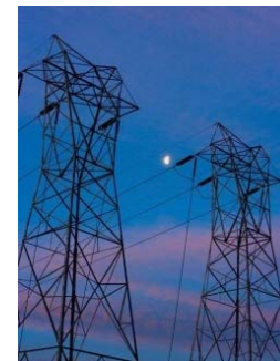
Transmission and Distribution Project
